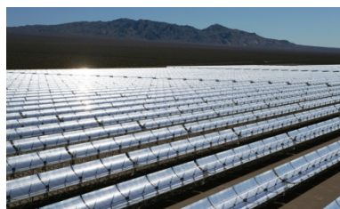
Large scale solar thermal (64MW), Nevada desert.
