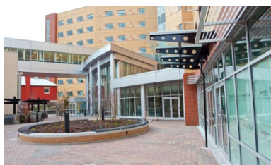
Sustainable design excellence, 500 bed hospital, Canada
