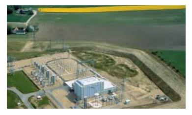
Station Kruseberg, Sweden, HV DC connection to Germany, 1994, 600MW, LCC
