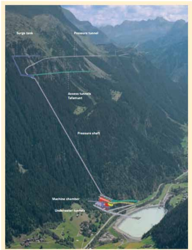
Course of the pressure water tunnel at the Kops II pumped storage power station (Fig.: Vorarlberger Illwerke)
